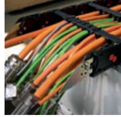
Program LC55: Wired with cables and connectors
