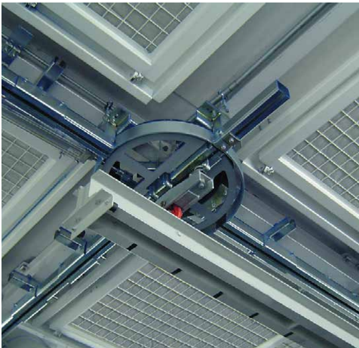
Combination of a turning switch and underslung crane with hoist
