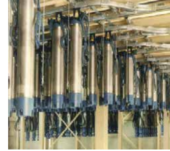
Overhead monorail system with buffer zone in a factory for submersible pumps
